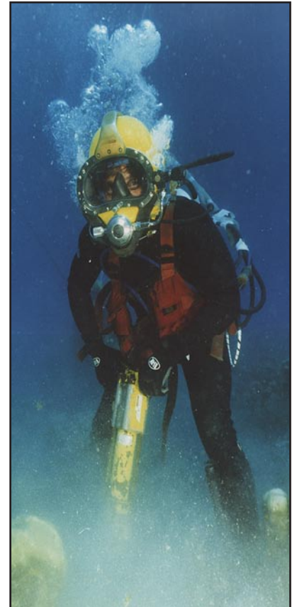
Figure 6-4. Underwater Construction Diving.
